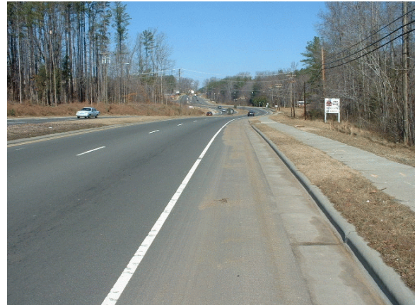
Figure 2. A wide 5 foot BL filled with sand.
